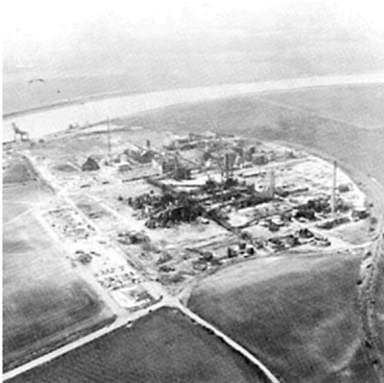
Figure A2.6 Works of Nypro (UK) Ltd at Flixborough after the explosion – 1 (R.J. Parker, 1975) (Courtesy of HM Stationery Office)
