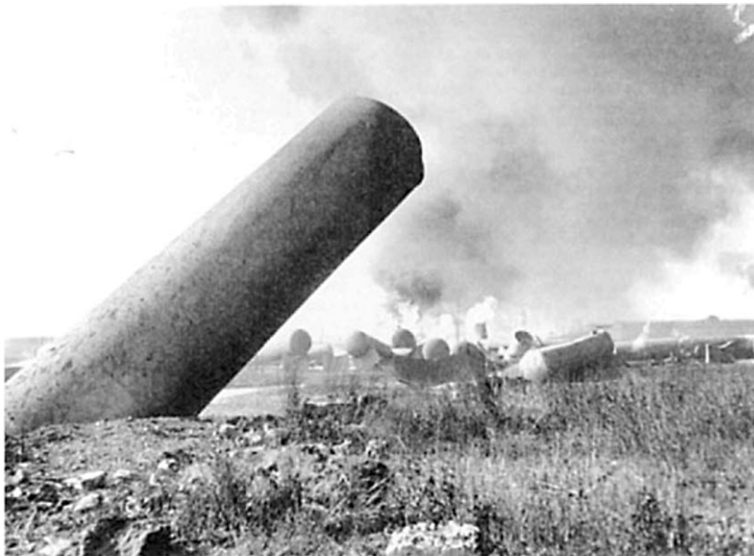
Figure A1.5 Port Newark, 1951: tank section part buried in ground (The Bettman Archive)
