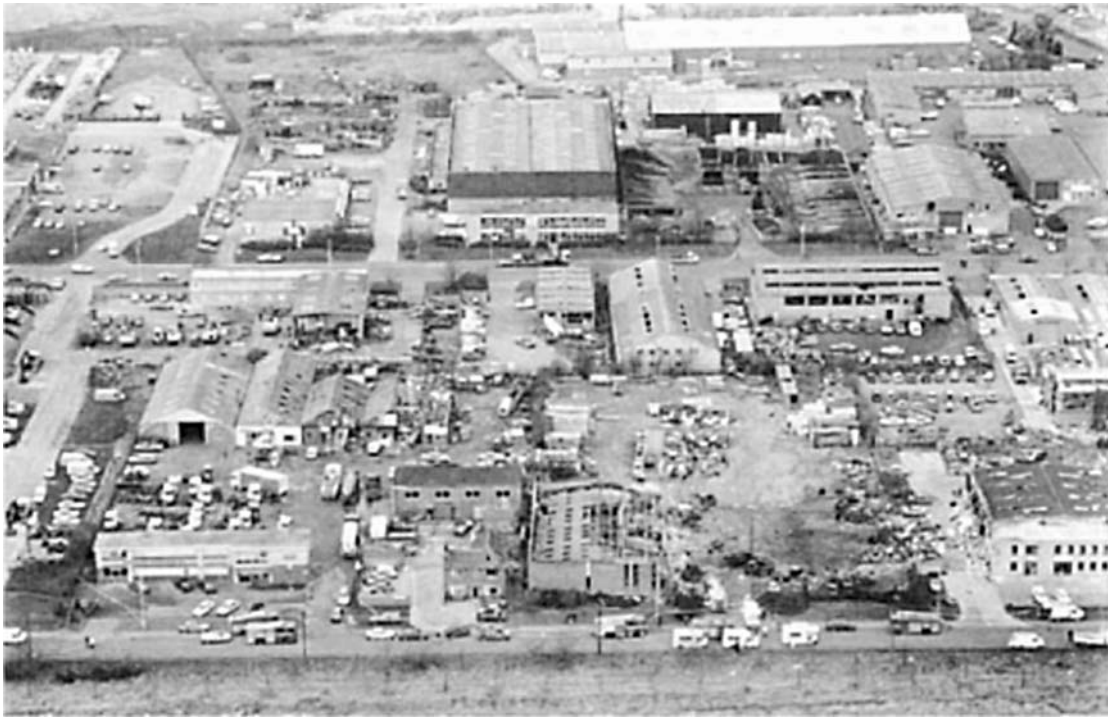
Figure A1.18 Peterborough, 1989: Vibroplant works yard after the explosion (Courtesy of the Peterborough Evening Telegraph)
