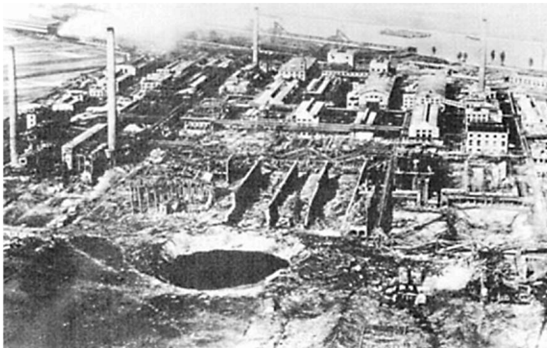
Figure A1.3 Oppau: BASF works after ammonium nitrate explosion, 1921 ( Badische Anilin und Soda Fabrik )
